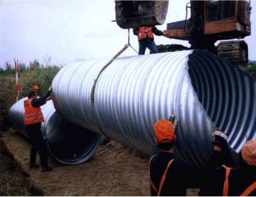
Picture 8. Three pipes used to build a culvert alt.1/ Corrugated steel pipe (CSP) galvanized alt.2/ Corrugated steel pipe (CSP) in trenchcoat alt.3/ Reinforced concrete pipes (RCP)
