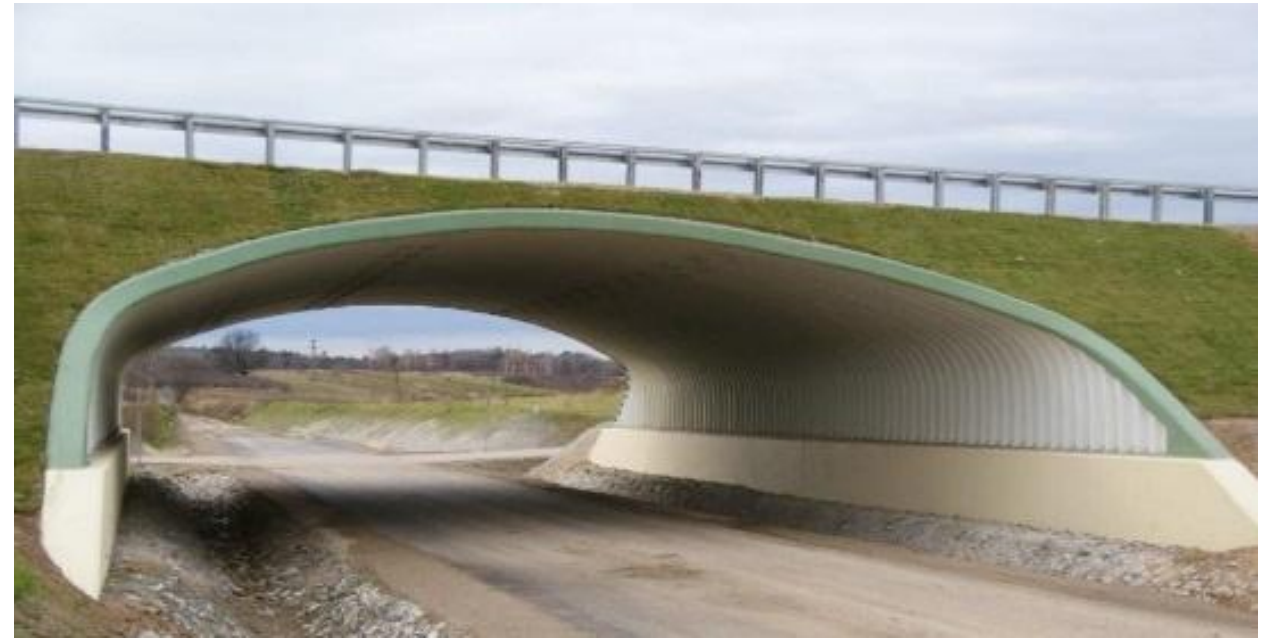
Picture 5. Two bridges having the same function concrete and buried corrugated steel bridge
