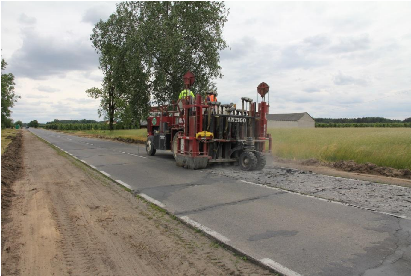
RUBBLIZING, Multi Head Breaker MHB
