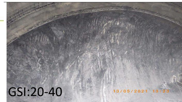
Rysunek 1. Fig. 1: overview face, serizitic and graphitic schists. Ground types O2 (-O3).
