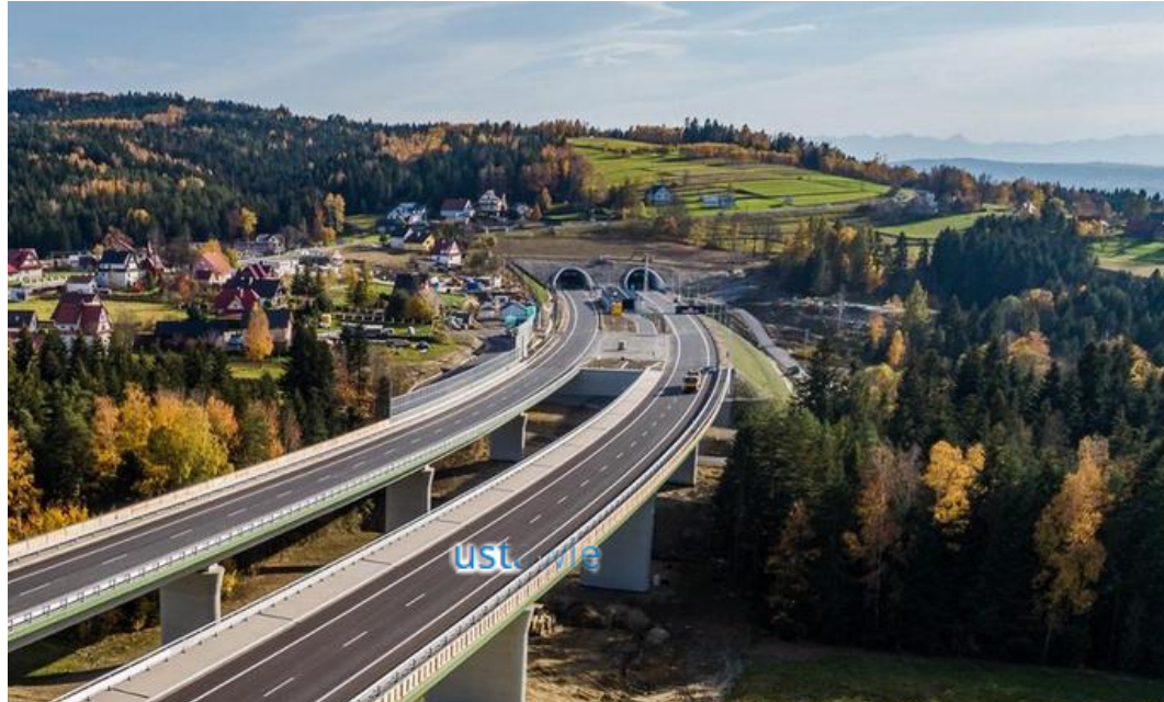
Tunel na Zakopiance S7 (ADECO-RS)
