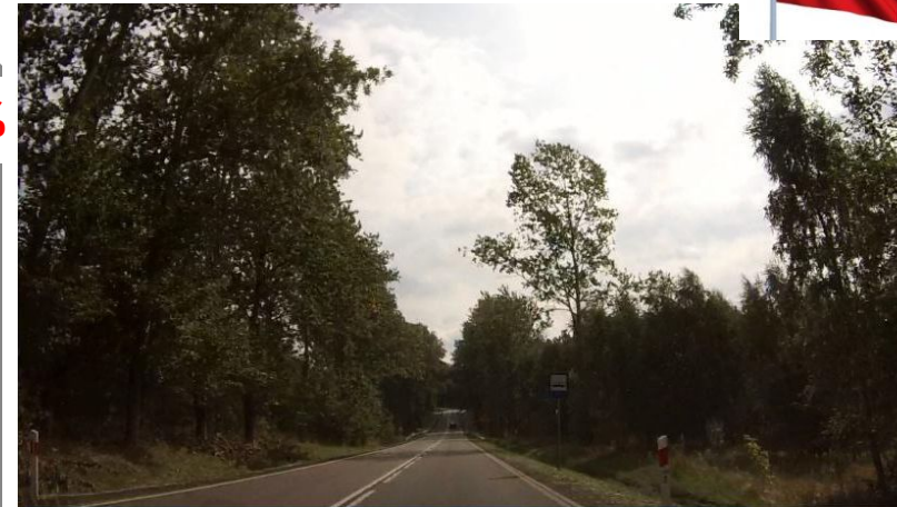
Inadequate shoulder width Score: High
