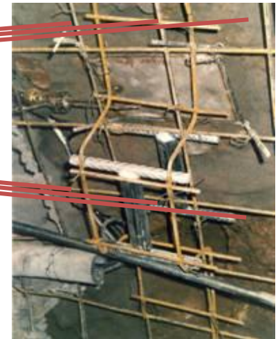
Strainmeters Pressure cells
