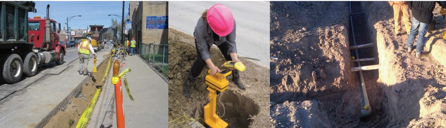
Left to right: Placement of 3M™ EMS Path Locating Tape over a gas pipeline.; Placing and mapping a 3M™ RFID Marker at a street crossing.; Placement of RFID markers at utility crossings and in change of directions and fittings is an excellent application.; EMS path marking tape and RFID ballmarkers complement each other for marking both the path of a facility and points of special interest.
