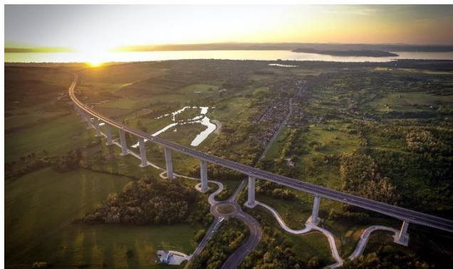
Kőröshegy Viaduct on M7 motorway
