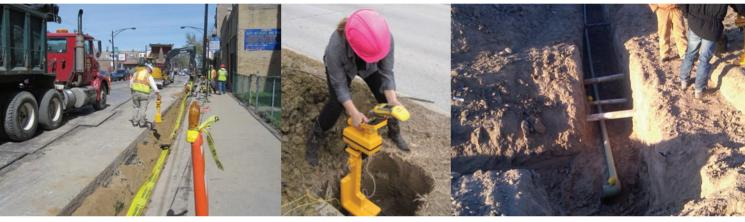
Left to right: Placement of 3M<sup>TM</sup> EMS Path Locating Tape over a gas pipeline.; Placing and mapping a 3M<sup>TM</sup> RFID Marker at a street crossing.; Placement of RFID markers at utility crossings and in change of directions and fittings is an excellent application.; EMS path marking tape and RFID ballmarkers complement each other for marking both the path of a facility and points of special interest.
