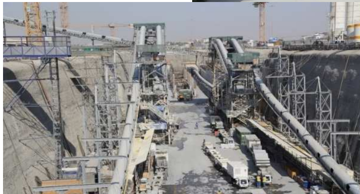
segments transport to TBM by Multi-Service-Vehicle (MSV)
