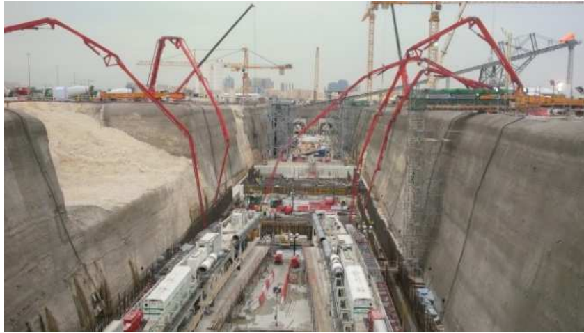
pull through of TBMs during excavation and concrete works in the station
