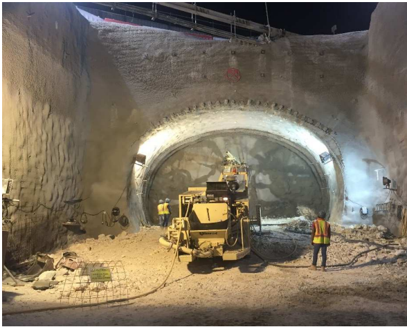
Shotcrete unit Normet 7110WPC- import from Europe Shotcrete C20/25, J2 early strength
