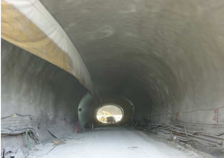
Underpass at Hamad Hospital Station
