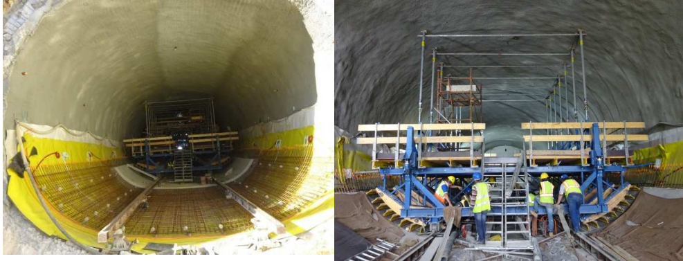
Invert - waterproofing, reinforcement, formwork & concrete at UP Hamad Hospital
