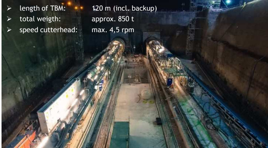
TVM S-844/845, TBM launch, Al Shaqab, 18.10.2015
