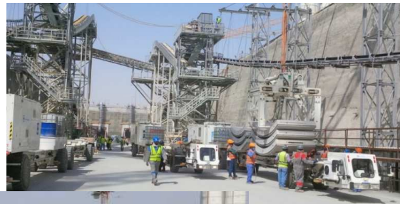
segments transport to TBM by Multi-Service-Vehicle (MSV)
