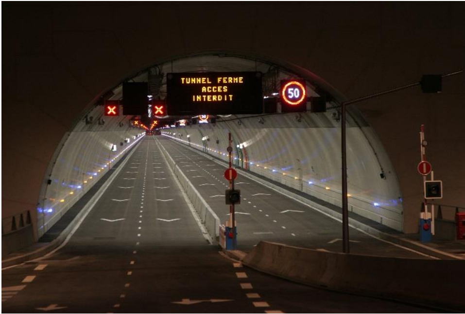
New road traffic tube, two lanes each direction, with a central crash barrier
