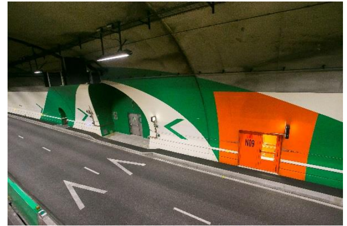
Emergency exit signage.
