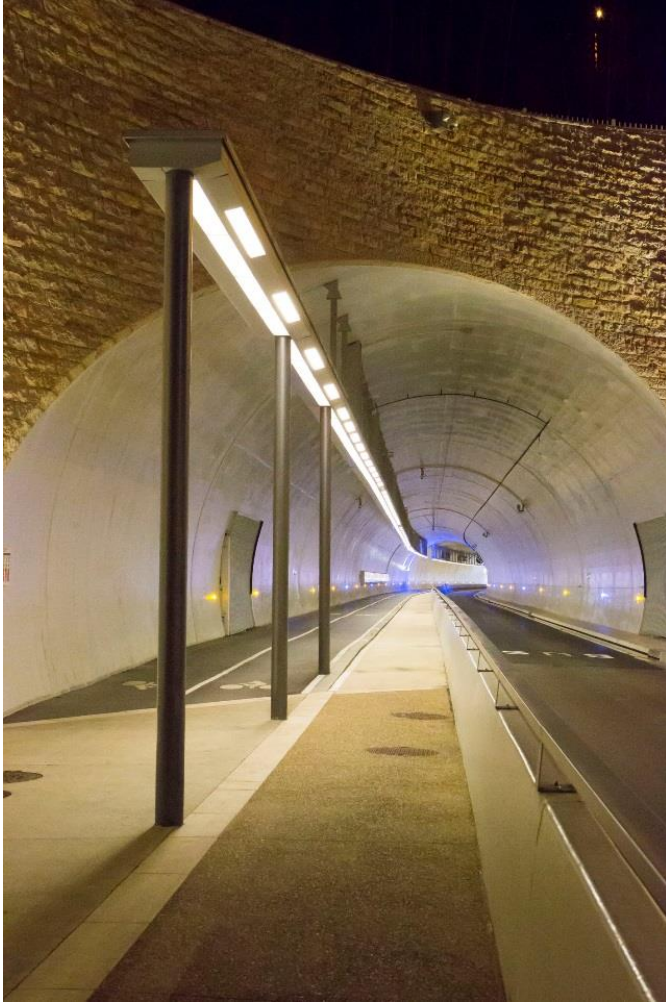
Overhead strip lighting
