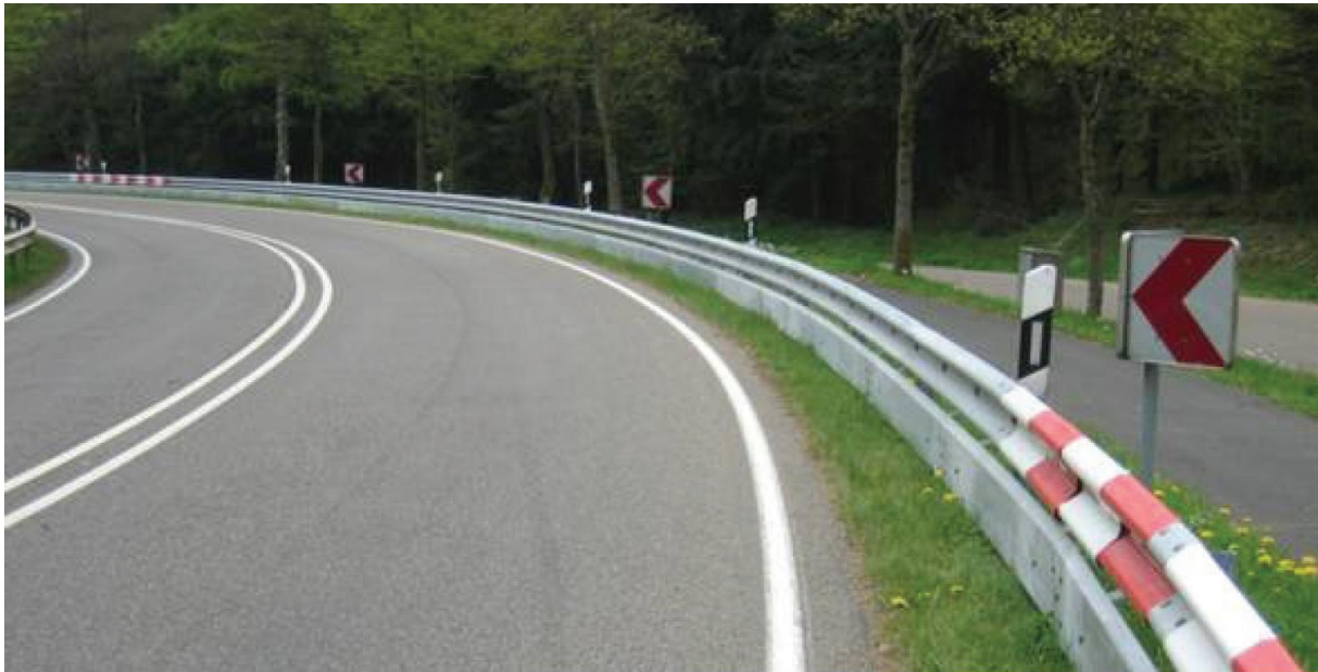
Figure 2 – Steel guardrail with MPS system
